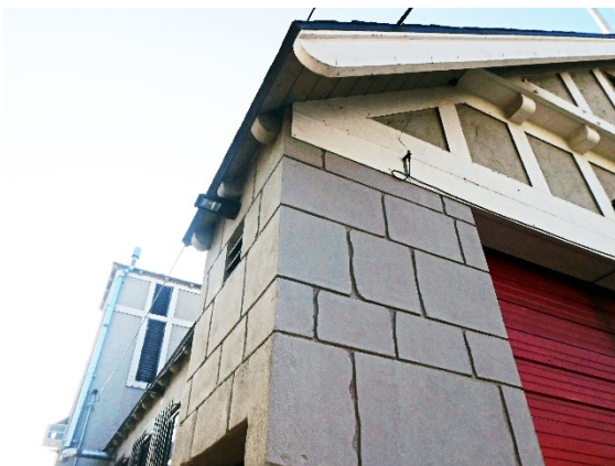
Figure 29: Detail of faux ashlar exterior finish, view of northwest corner (GPA, 2019)
