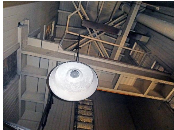
Figure 28: Top of hose tower, showing walking platform, metal pipe railing and hose rolling mechanism (GPA, 2019)
