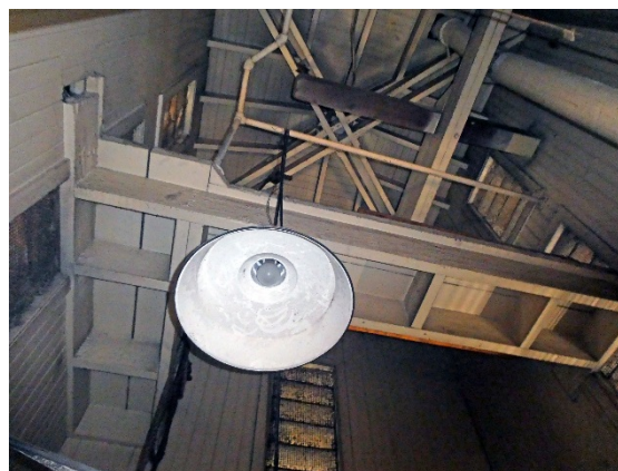
Figure 28: Top of hose tower, showing walking platform, metal pipe railing and hose rolling mechanism (GPA, 2019)
