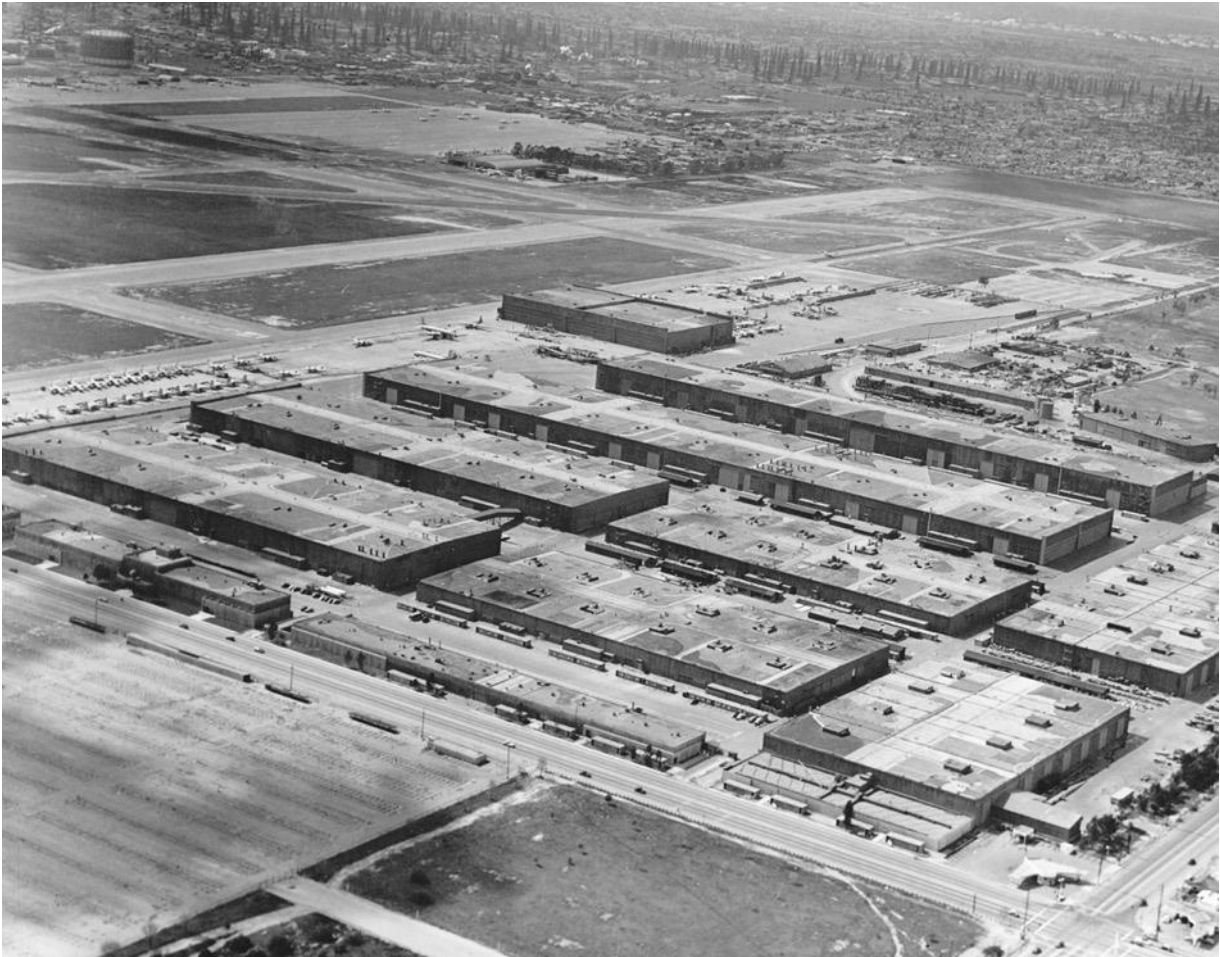
Fig. 65. Aerial view of the Long Beach Douglas Aircraft plant, 1941. The new plant was 1.4 million square feet of assembly space and eleven buildings on parcels purchased from the Montana Land Company adjacent to Long Beach Airport. The new assembly plant construction was funded mostly by the federal government and was the first air-conditioned factory complex in the U.S. It was designed without windows so it could operate 24-hours a day during World War II blackout conditions. This new plant was like a city within itself that included a system of streets laid out to reduce congestion and to accelerate the flow of materials and labor operations.
