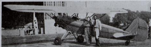
Mr. Aikens is shown standing beside his Meteor High Wing Mono-plane, powered with a 100 H.P. Kinner motor. Cruises at 110 MPH. Top speed, 135 MPH.
